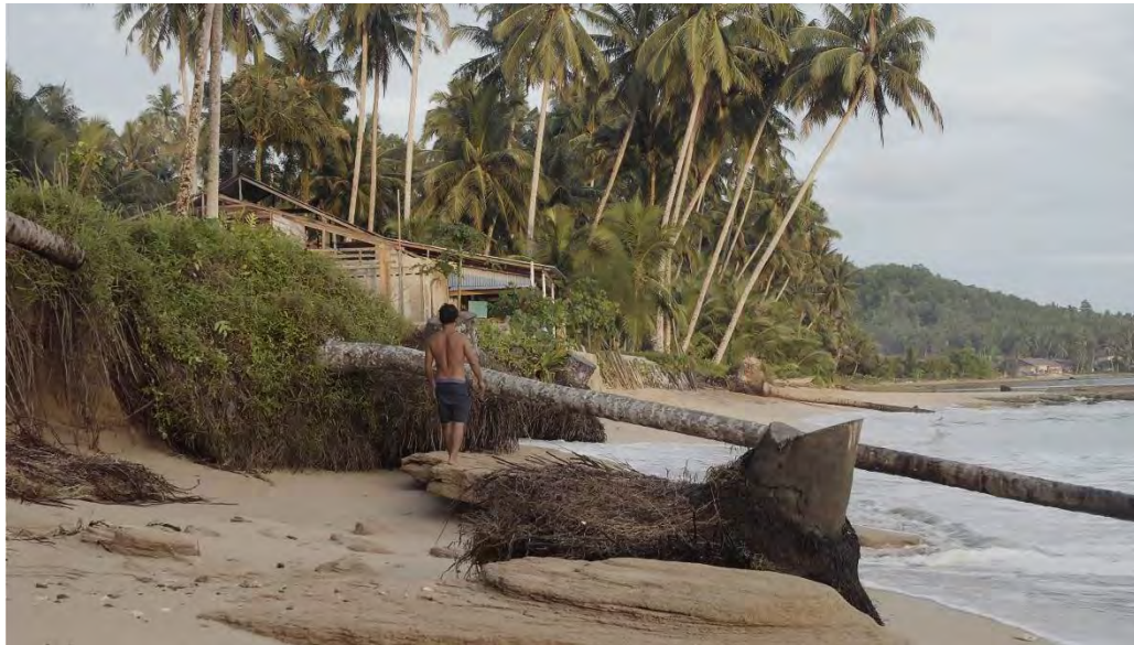
Figure 30: Aprianto returns home – note how far the tide comes in, and the extent of erosion and fallen debris
